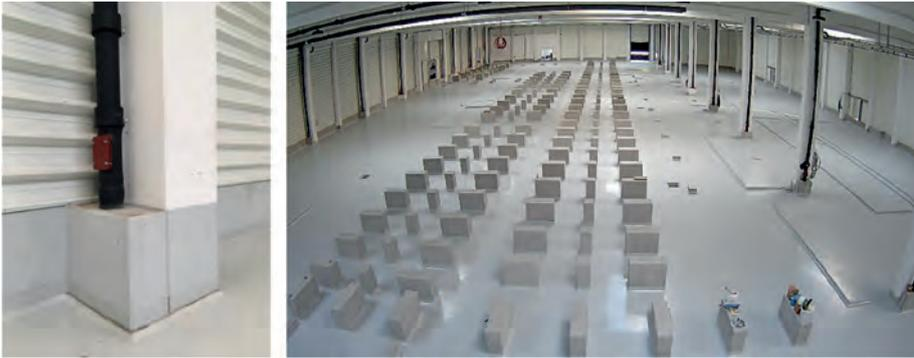
**Fig. 4: Indoor installed rainwater downpipes securely embedded in concrete up to the maximum expected water retention level**
